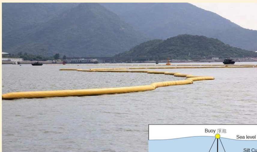
淤泥屏障 Silt curtains
